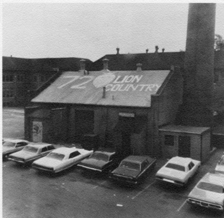
This is Lion country!!! Thanks to the brave souls who risked their lives to paint the roof of the powerhouse.
